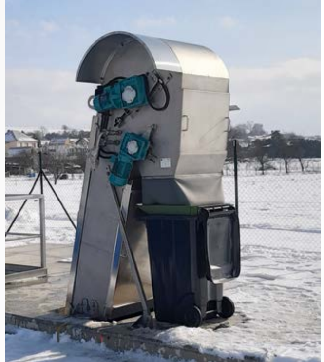
Pumping station, Sazovice, Czech Republic, 1000_CP_3250_Z
